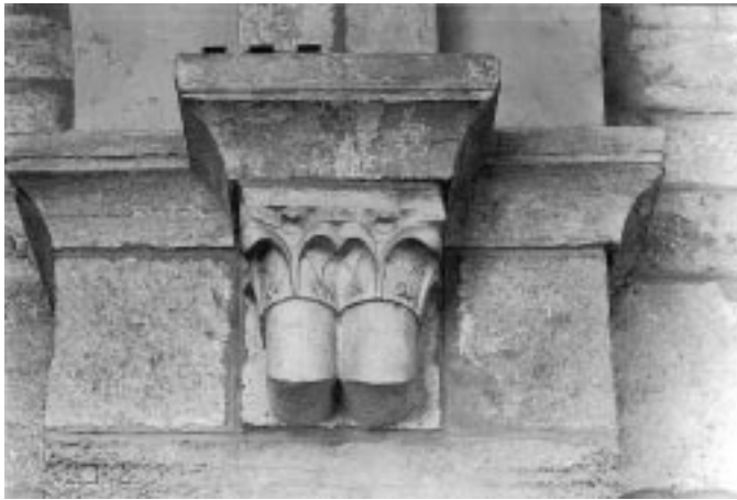
Fig. 13: Elbow columns (No. 11), portico, al-Aqsa mosque, Jerusalem (Courtesy of Israel Antiquities Authority).
