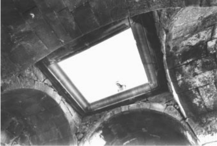
Fig. 15: Umm Idj-Djimal, the "Praetorium". Note the moulded square frame, once roofed by a dome.
