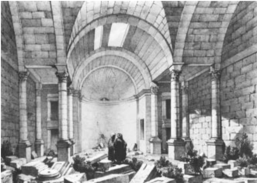
Fig. 5: Musmīyah, a Temple, general view of the naos towards the adyton. Note the "Reconstructed Roof" (drawn by de Laborde in 1827).
